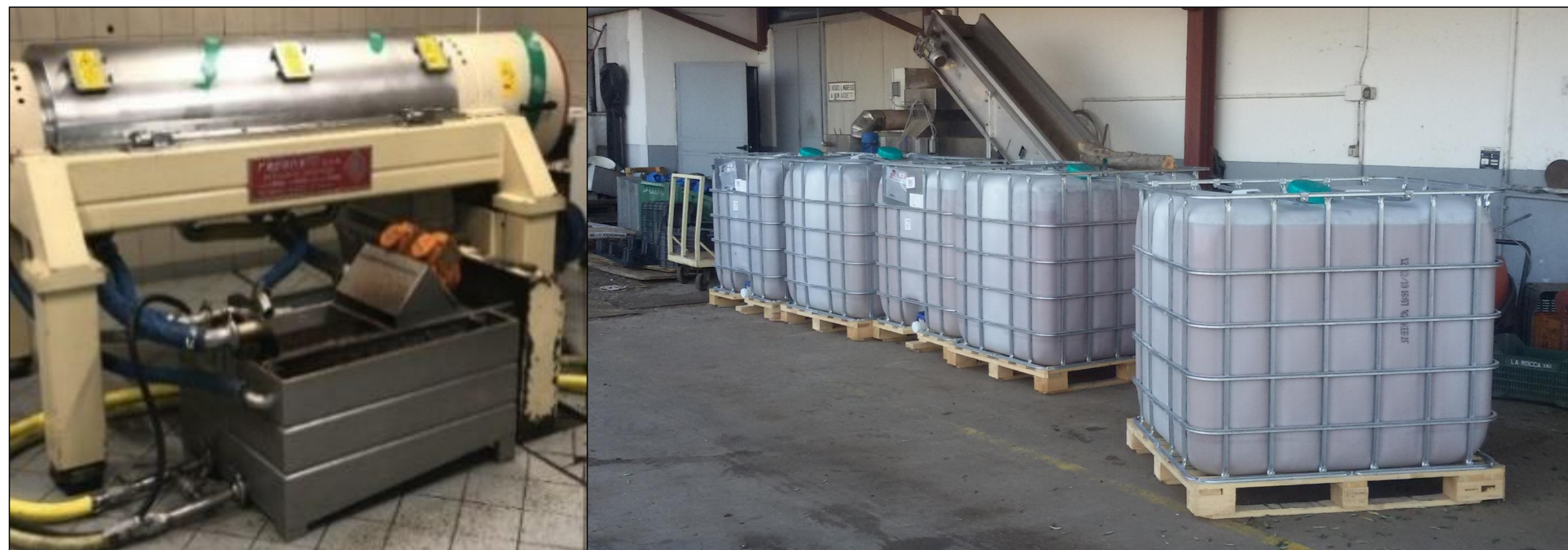
Olive oil production plant
