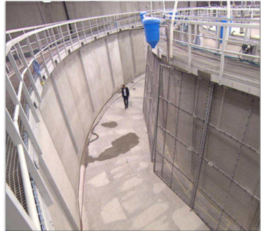
Final construction phase RAS2020
